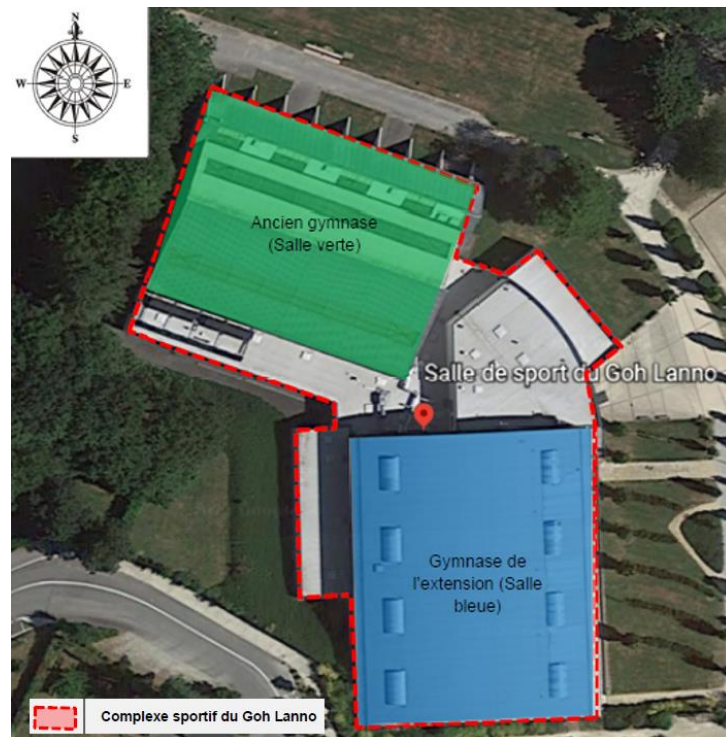
Figure 13: photos du site
