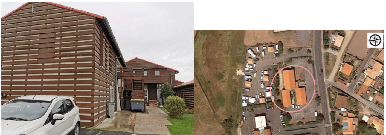
Figure 10: photos du site
