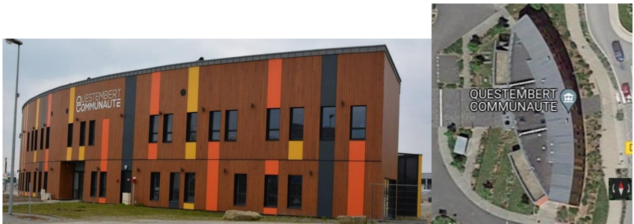
Figure 12: photos du site
